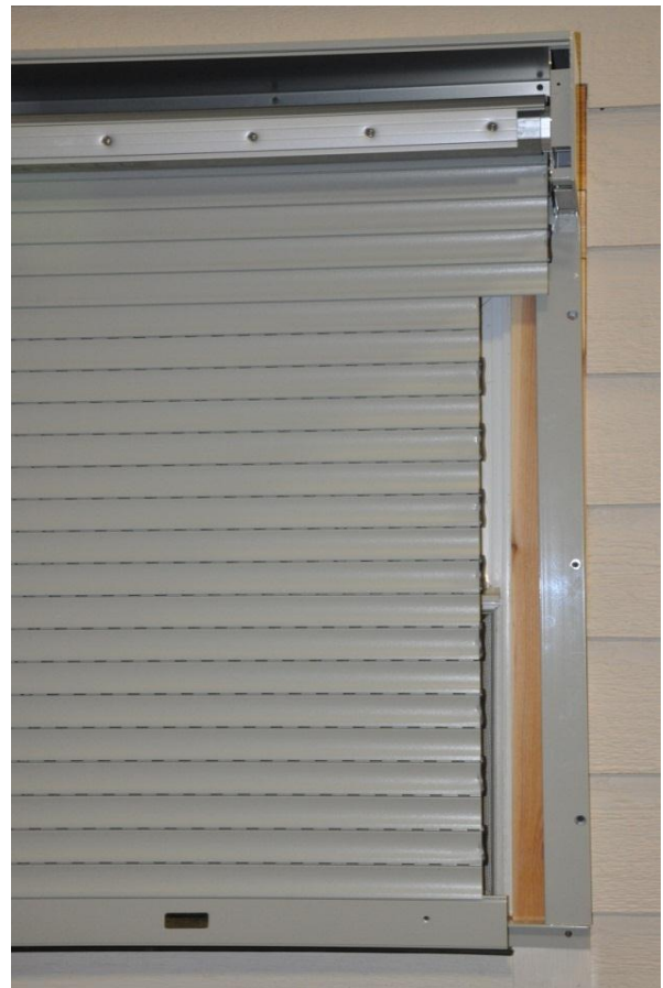
13. Unwrap slat from axle and hang outside of rails. Attach balance of slat bundle and raise shutter with crank.
