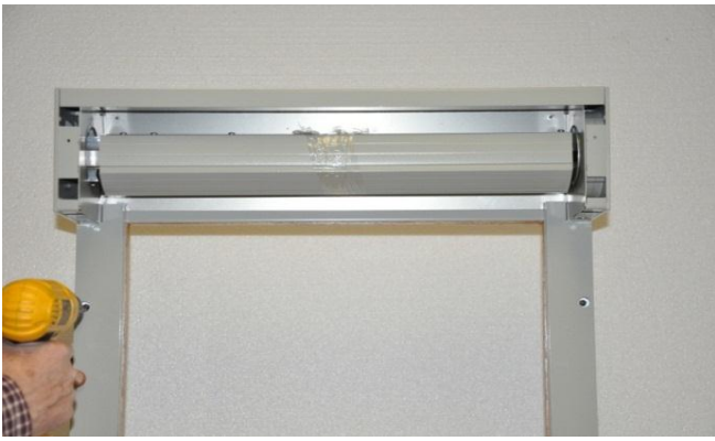
10. Attach the rails to the wall.
