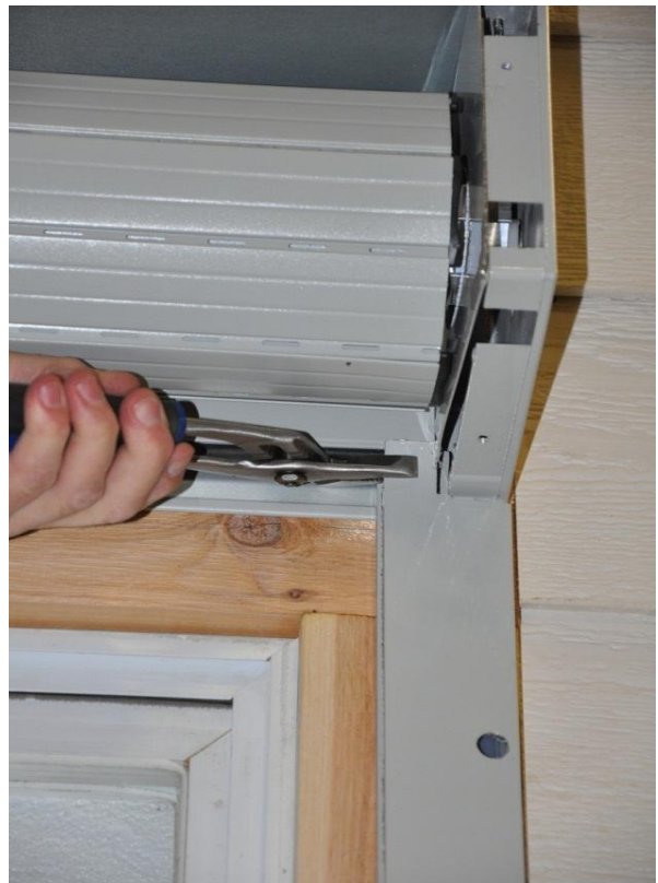
15. Form front rail guide. Use channel lock pliers to bend front ear of rail forward 30 degrees. This forms guide for slat to flow into rail. Lower shutter to check operation.
