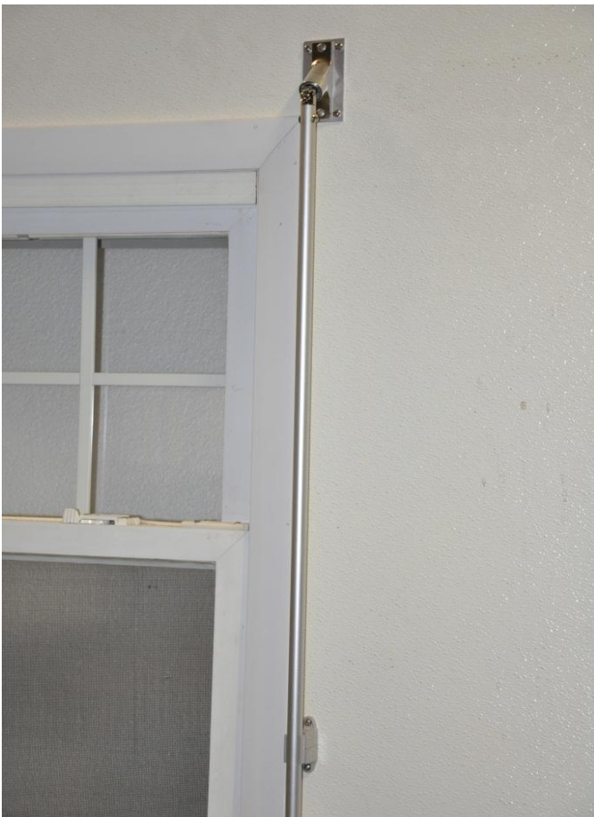
12. Attach crank universal bracket to wall and check operation.
