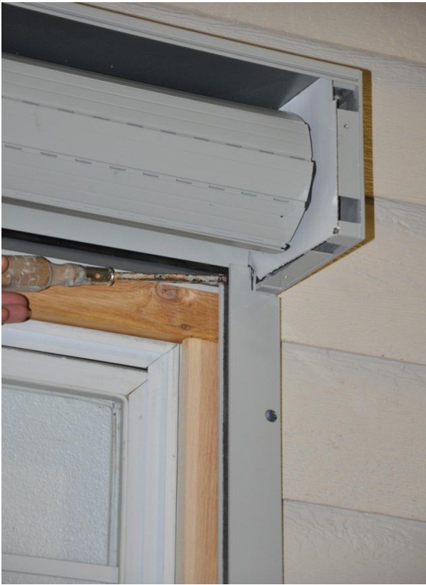
14. Form side guide of rail by Pushing top sideways 1/8" .
