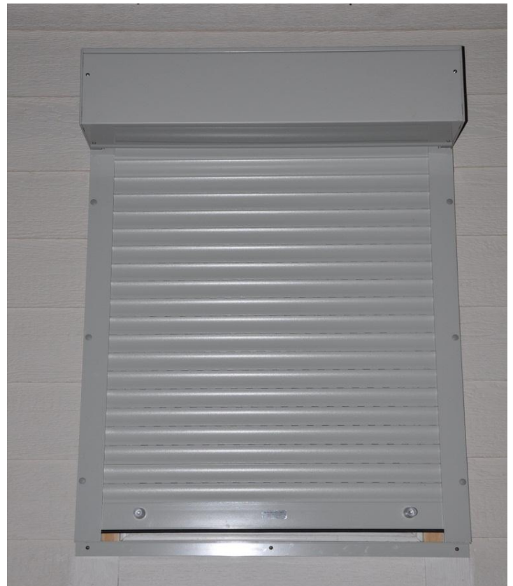
17. Install face cover and seal top and side of box to prevent leaks.
