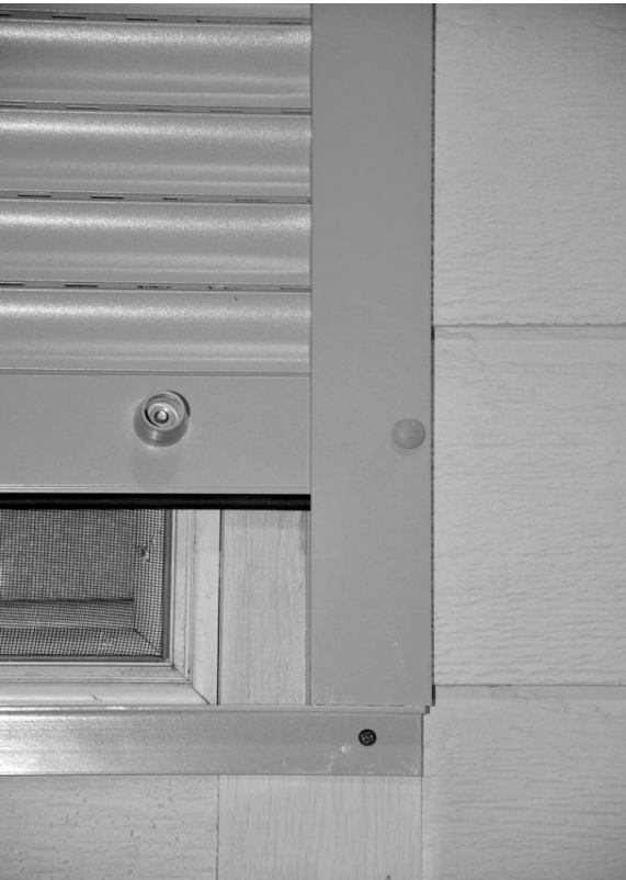
16. Install stops on base slat so shutter cannot be rolled in box cover and install plug buttons.
