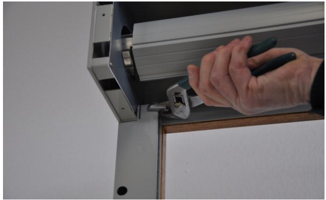
12. Form front rail guide. Use channel lock pliers to bend front ear of rail forward 30 degrees. This forms a guide for the slat to enter the rails.
