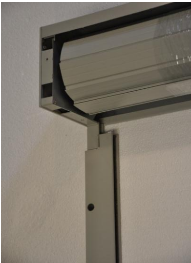
3. Slip rails onto end cap locator legs.
