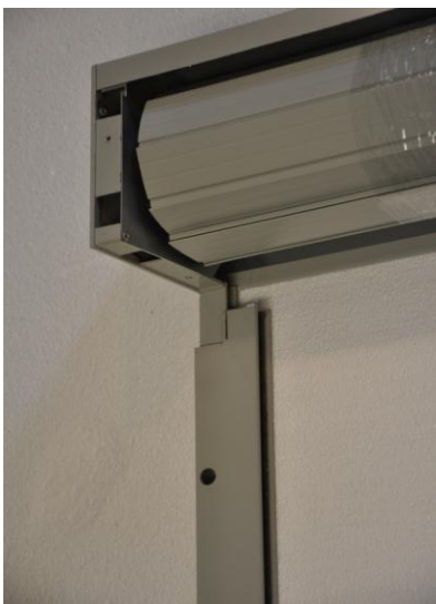
3. Slip rails onto end cap locator legs.
