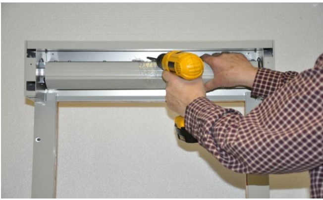
5. Set rails and storage box to the wall location. Always support box until attached to wall or the locator legs can break. They are not load bearing.
