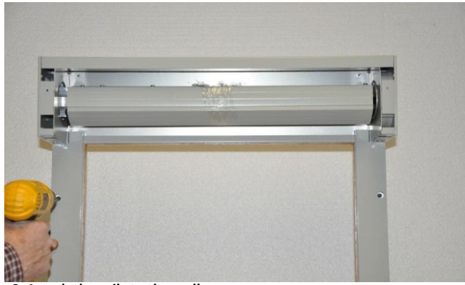
6. Attach the rails to the wall.
