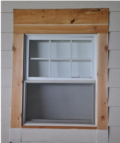
1. Add trim to side and top of windows flush to outer surface of window frame and any other extension. Shutter needs to be mounted on a flat surface.
