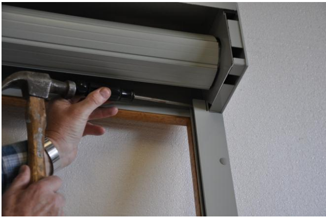
11. Form side of rail by pushing top sideways 1/8"
