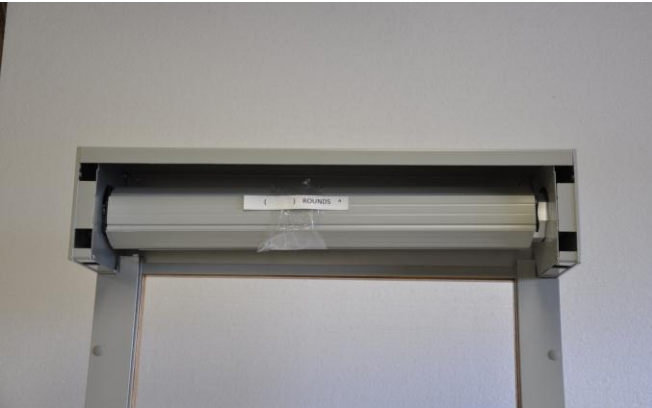
7. Attach motor wire to switch and connect to power. For installion, a short cord with plug can be used. One wire to connected to the white of the motor and the other touched to the black or red for up or down control.
