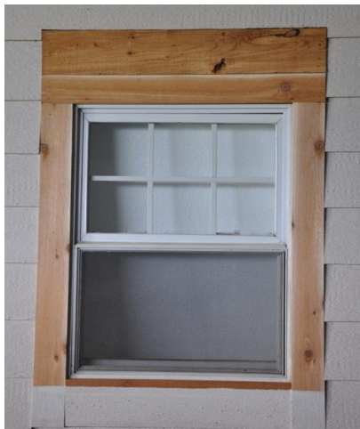
1. Add trim to side and top of windows flush to outer surface of window frame and any other extension. Shutter needs to be mounted on a flat surface.
