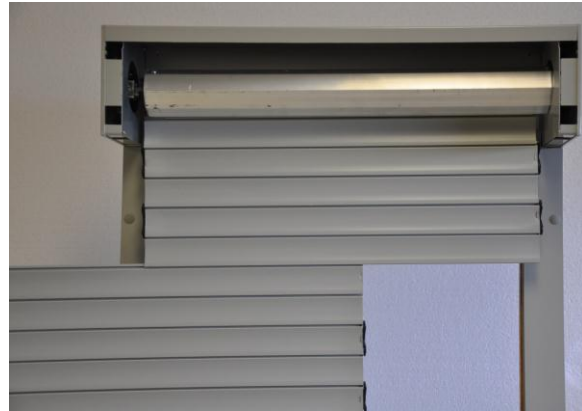
8. Unwrap slat from axle and hang outside of rails. Attach balance of slat bundle and raise shutter.
