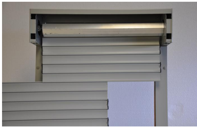
8. Unwrap slat from axle and hang outside of rails. Attach balance of slat bundle and raise shutter.
