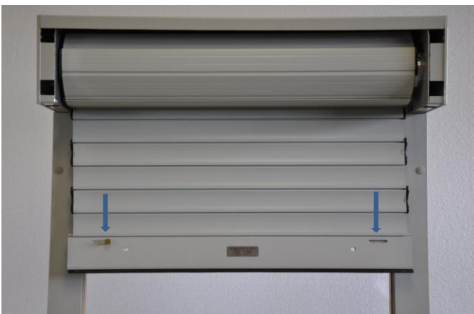
9. Remove dead bolts if installed and raise shutter completely. Lower slat into rails.
