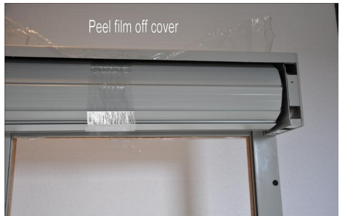
2. Remove protective film from box covers.
