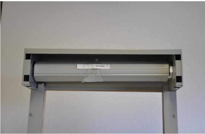
7. Spin axle in direction of shutter going down ( ) turns. Number of turns depends on shutter height. Check information on shutter roll. Turning the wrong way will cause torsion spring to detach.
