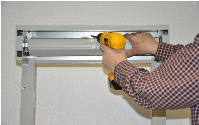
5. Set rails and storage box to the wall location. Always support box until attached to wall or the locator legs can break. They are not load bearing.
