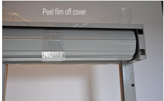
2. Remove protective film from box covers.
