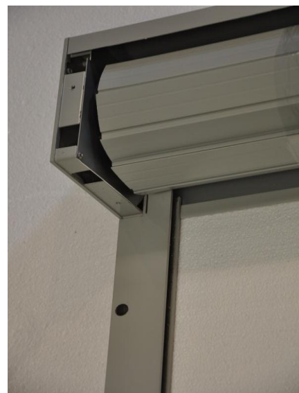
4. Rail totally on locator leg.
