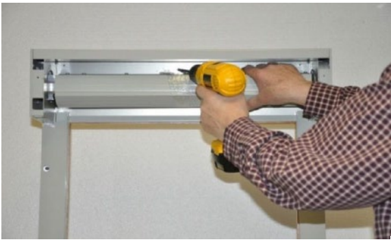
9. Set rails and storage box to the wall location. Always support box until attached to wall or the locator legs can break. They are not load bearing.
