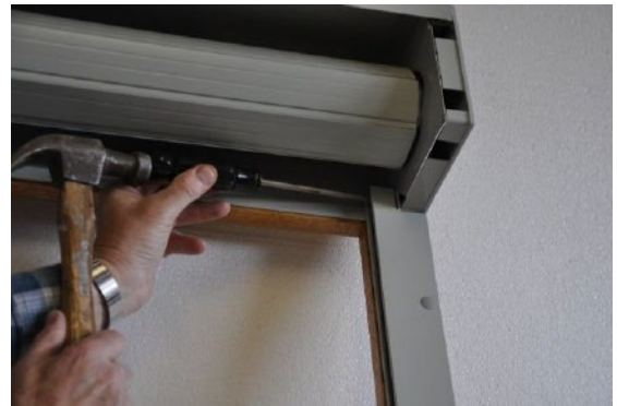
With large screwdriver and hammer push side ear to side about 1/8".
