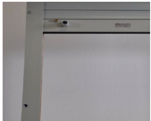
Install plug buttons into track holes.
