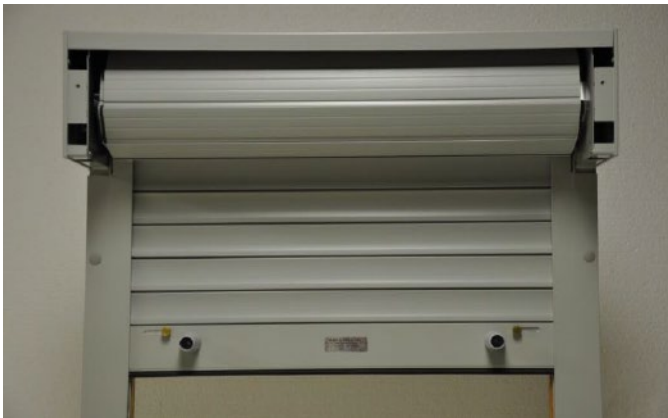
Attached stops to base slat so shutter does not go up into the coil box.
