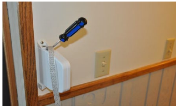
Attach strap recoil inside and pull out all the strap as far as it will go and lock in place.
