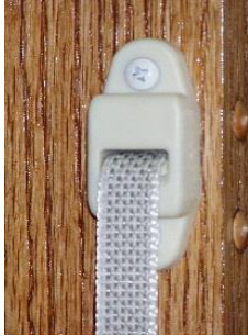
Put strap through wall bracket and put strap through wall to connect to outside reel. Tape strap to hex saw blade or wire and push through wall.
